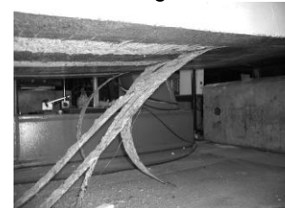
Failure mode for slab No.5, breakage of fibre and debonding of the sheet
